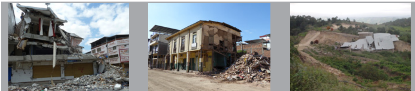
Examples of some of the damage observed in Manta, Portoviejo and San Isidro (left to right)
