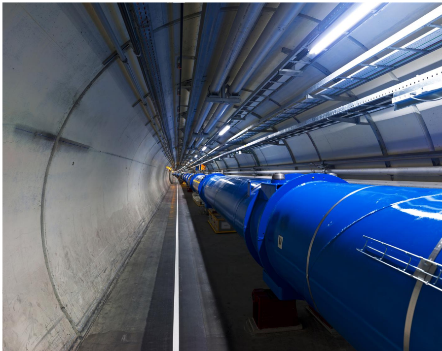
Figure 3.1: Interior of the 3.8 m diameter LHC tunnel between the ATLAS and ALICE experiments. [26]
