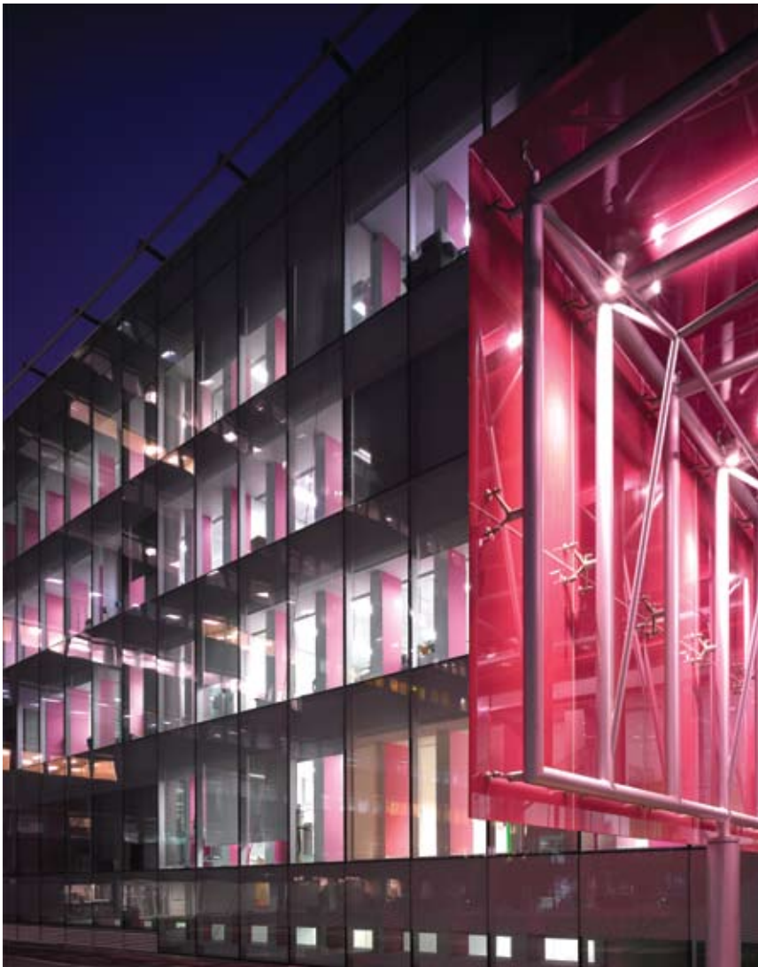
Night, camera, action! Stunning images of the South Kensington Campus, taken by renowned architectural photographer Christian Richters, are now available from the College's digital image library. Visit https://imageslib.cc.ic.ac.uk and search for 'buildings at night'.
