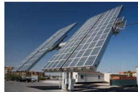
A photo of Amonix Concentrator Photovoltaic System at the University of Nevada, taken on one of Professor Ekins-Daukes’ field trips.
