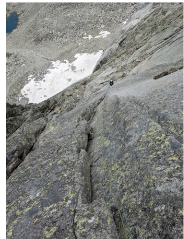
Figure 3.10: Cracked slabs of the Peigne.
