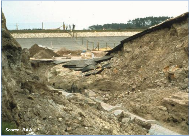
dam breach at crossing with underlying water transport pipe after flooding of a new canal section
